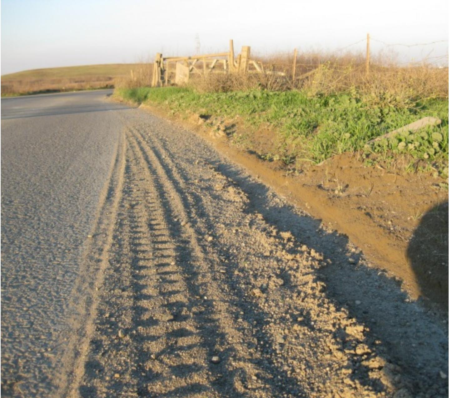
Above image shows contaminated soils along Portrero Hills Lane public access road to the Landfill. All the dirt on the shoulder above the road surface is sediment run off from the landfill.
